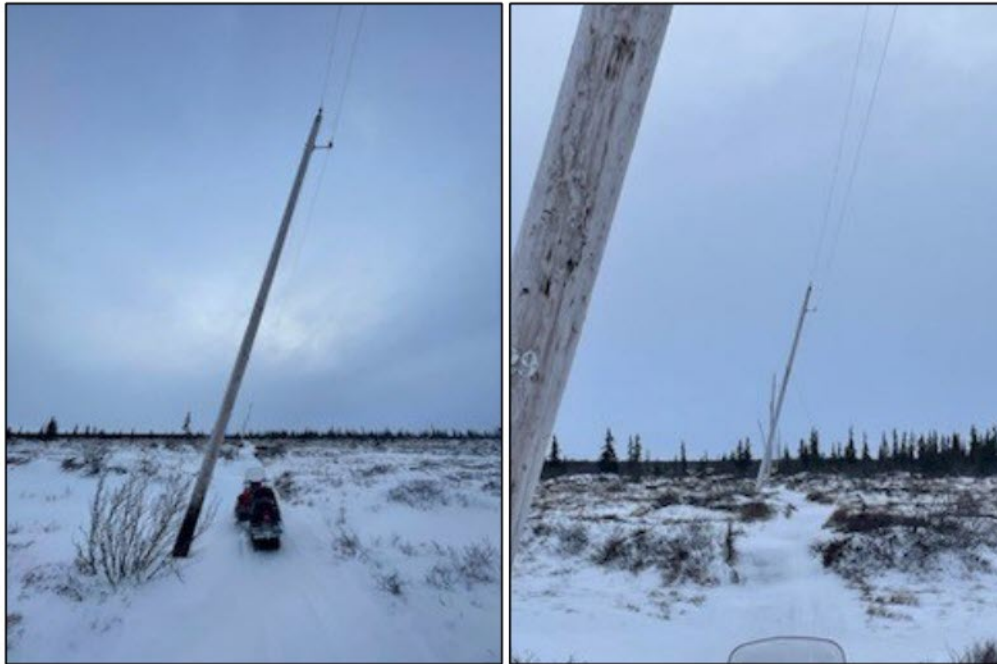
Pictures of leaning poles and distribution lines in Oscarville
